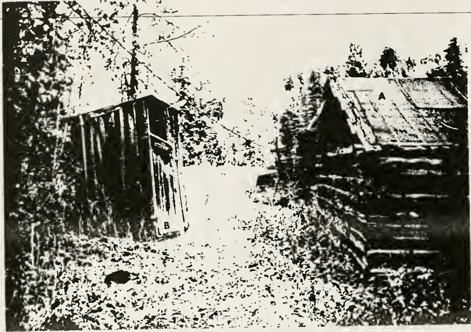
Figure 79. A. Structure #31 B. Structure #32 (north view)
